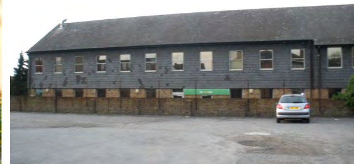
Former stable and brew house, now much altered, 820 Uxbridge Road
