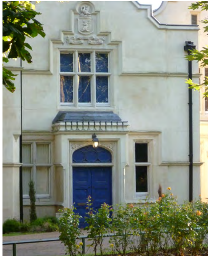
Barra Hall front door
